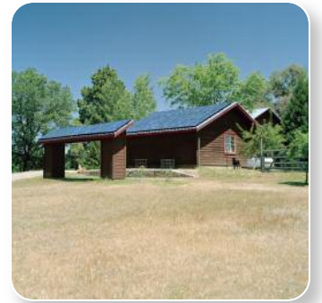
GE PV Modules – Home Installation Placerville, CA
