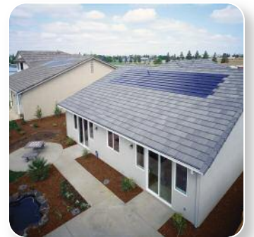
Roof-integrated Panels Sacramento, CA
